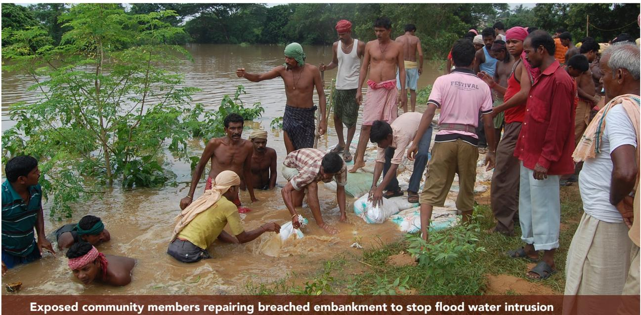
Exposed community members repairing breached embankment to stop flood water intrusion
