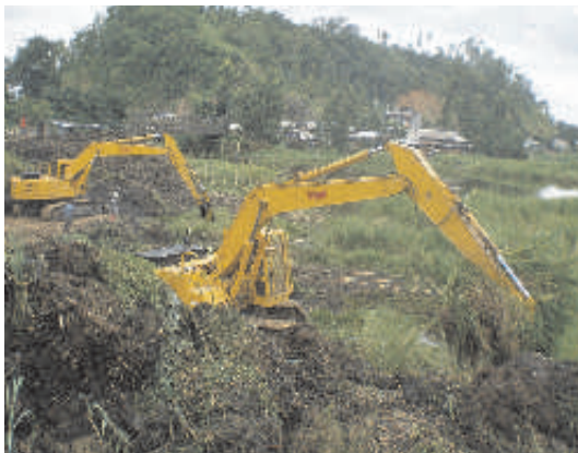
Phumdi removal with excavators
